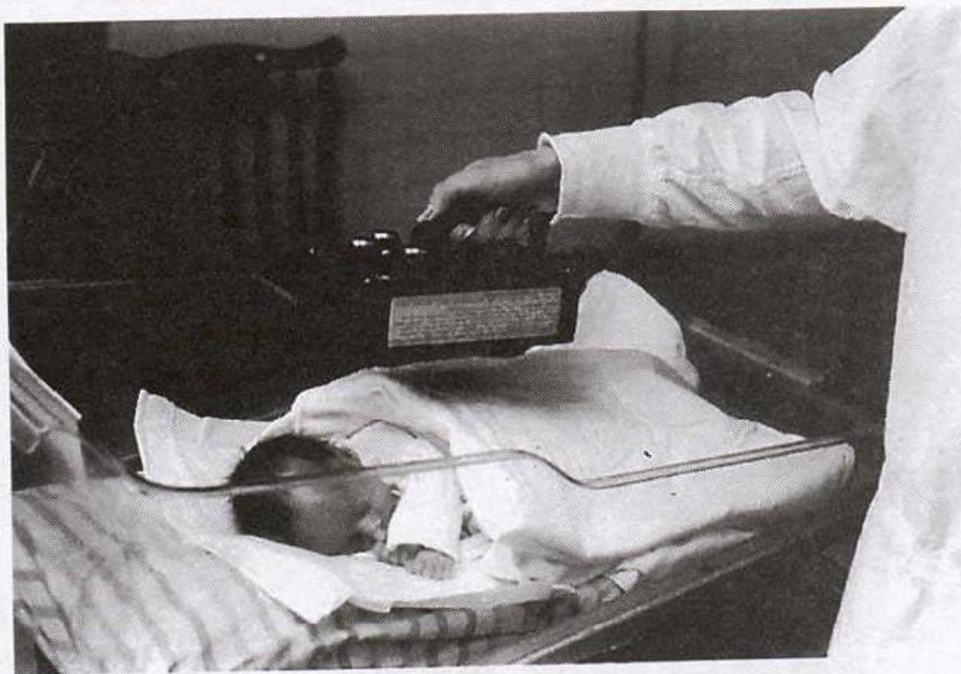
FIGURE 1-1. A specially designed battery-powered infant hearing screener used in the early 1960s known as the Apritron (from the auro-palpebral reflex, the involuntary body movement and eye blink resulting from sudden sound onset). The examiner presented a sudden onset narrow-band noise stimulus of 90 dB SPL followed by observation for the presence or absence of reflexive infant responses.
